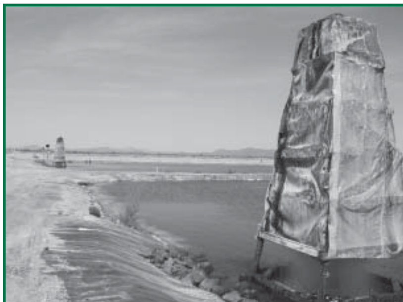
Figure 1. An aeration tower at Arizona Mariculture Associates. The tower contains multiple layers of screened plates which de-gas nitrogen from the supersaturated pumped groundwater, while increasing its oxygen content, as it falls through the screens.
